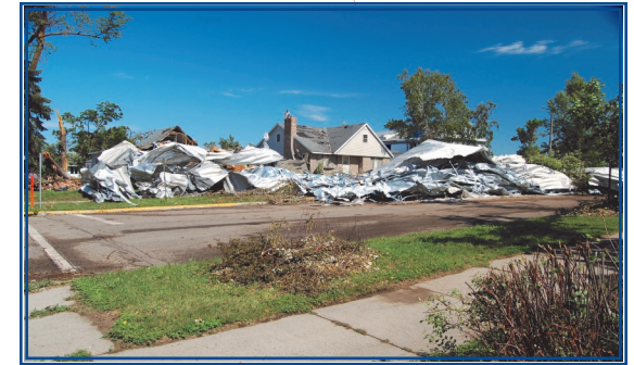
Wadena, MN an EF4 tornado struck on June 17th— The metal roof of the city community center was twisted and blown 4 city blocks! Photo courtesy of FEMA/Michael Mancino
